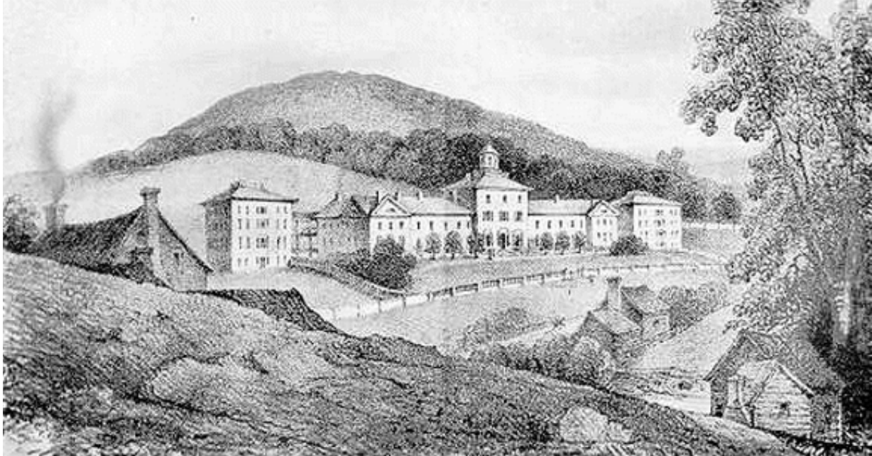
Image Three: Western Lunatic Asylum in Staunton, Virginia in 1837 showing the Kirkbride Linear Plan and ample grounds for patients. During the 1870s, superintendents at Central Lunatic Asylum proposed the construction of a new building for patients to be constructed in this fashion. The Annual Report of Dr. Francis Stribling, Physician of the Western Lunatic Hospital (Staunton, VA: Order of the Court of Directors, 1837).
